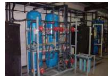
FIRE PROTECTION SYSTEM
